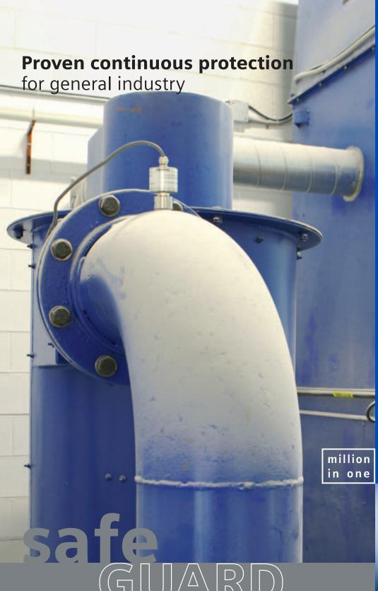
Process protection devices act as an early warning system to avoid costly process interruptions and equipment breakdown. SITRANS AS 100 reacts instantly to changes in solids flow to warn of blockages, product absence or equipment failure such as burst filter bags.
