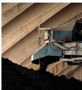
Monitoring throughput in mining production with Milltronics MSI belt scale
